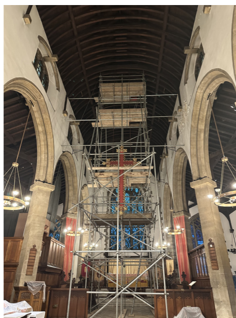
CHURCH UNDER REPAIR
