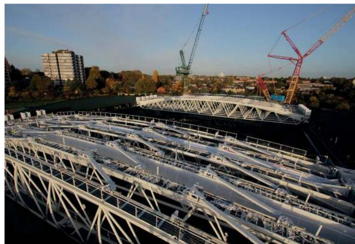
The view on top of No.1 Court- all trusses securely in place
